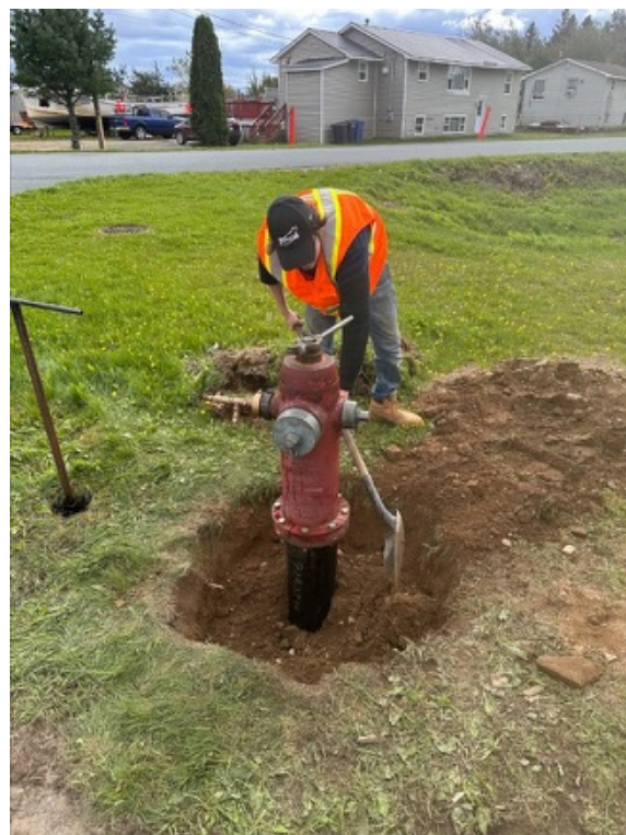
Esgenoopeitj Operator Raine Somerville completing hydrant maintenance.
